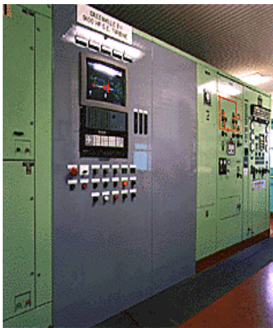
PLC-based integrated replacement controls with MMI graphic workstation for one GE Frame 3 compressor train
