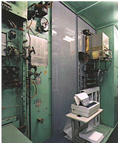
PLC-based integrated replacement controls with MMI graphic workstation for one GE Frame 3 compressor train
