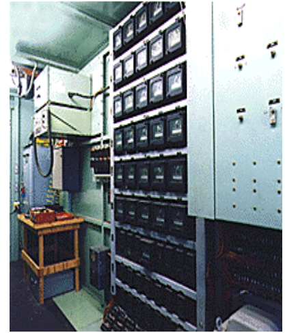
Existing 1960's electro-hydraulic, pneumatic, and relay-based controls for one GE Frame 3 Compressor train
