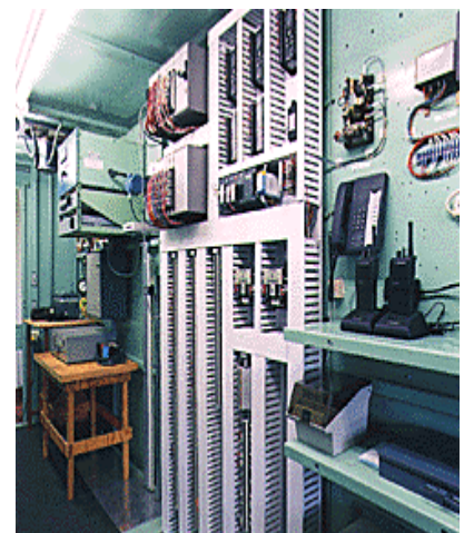
PLC-based integrated replacement controls with MMI graphic workstation for one GE Frame 3 compressor train
