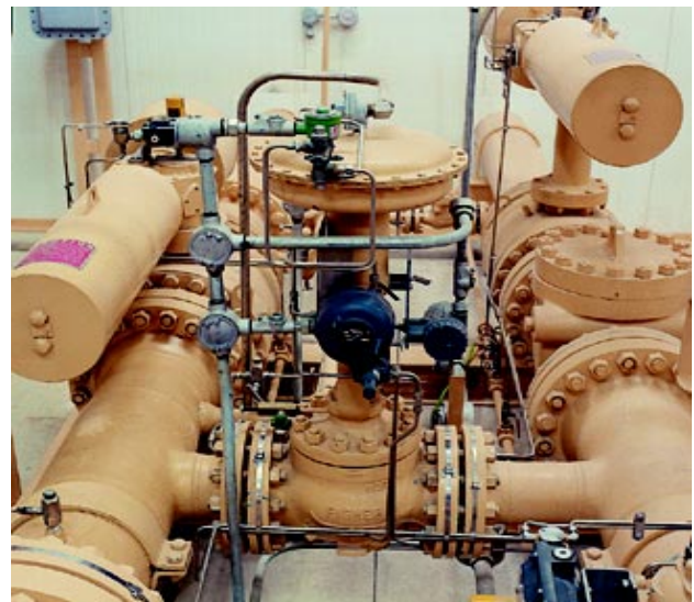
Installation of a Petrotech model RVAM compressor anti-surge recycle valve assembly
